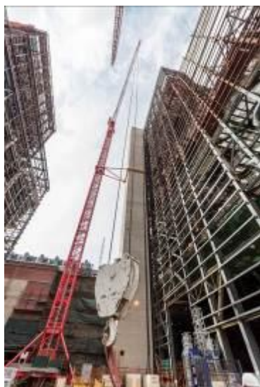
The WOLFF 1250 B with a 60 meter jib and a tower height of 120 meters is tied to stair tower of the boiler house with only one tie.
