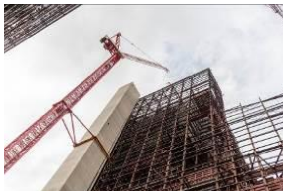
The WOLFF 1250 B with a 60 meter jib and a tower height of 120 meters is tied to stair tower of the boiler house with only one tie.
